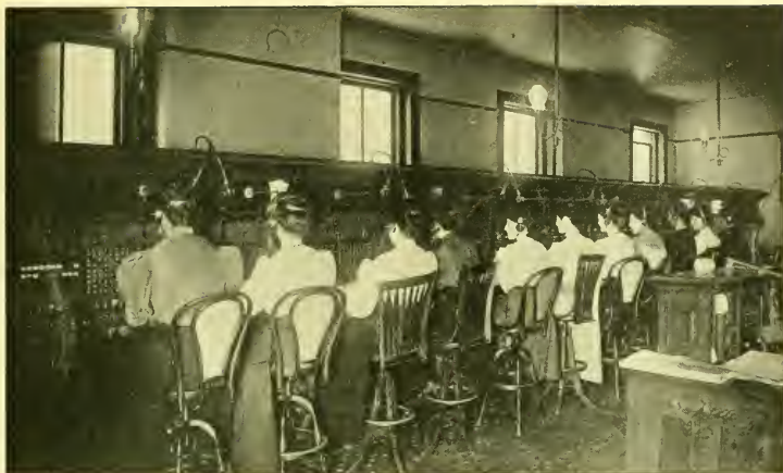
The Operators at the Switchboard.
